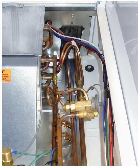
Glycol cases typically have a balance valve located in the outlet line inside of the case. If a stop solenoid is provided, it will also be located in the outlet line. Schrader valves are provided inside the case on the right-hand side of the coil for venting and draining the system.
