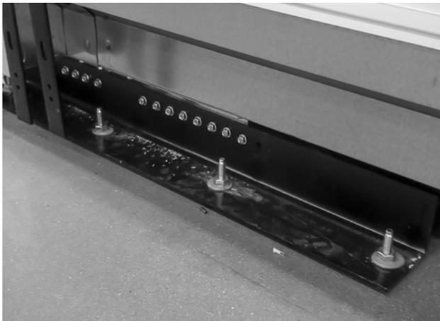
FIGURE 1: Holes Drilled for Rear Bracket
