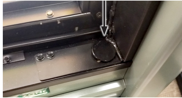
FIGURE 33: Torque Adjuster Plug
