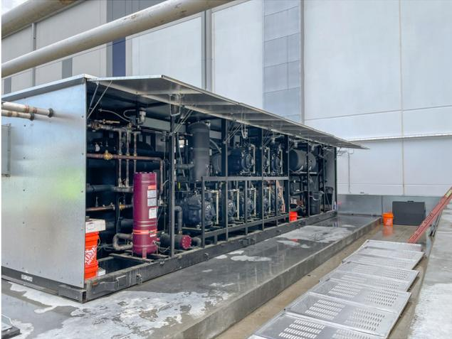
This project required two Zero Zone Genesys™ outdoor packaged racks. One rack is to keep the dock cool and has a refrigerant capacity to provide 60 tons of cooling. Half the capacity of the dock rack, along with another full rack with a capacity of 200 tons, were needed to cool the 120,000 ft<sup>2</sup> facility.
